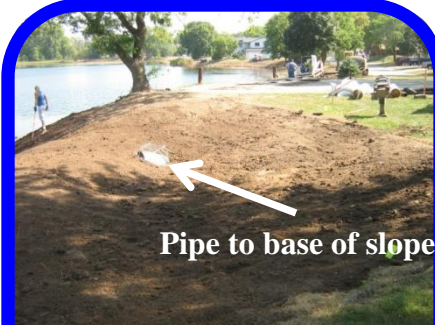
Slope drain installed at location of concentrated flow
