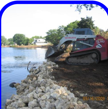
Imported granular fill behind weighted toe to match existing bank
