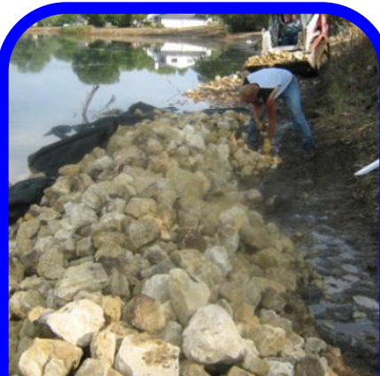
Installation of weighted toe at base of eroded slope
