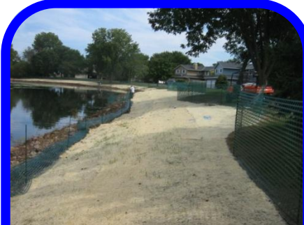
Seeded areas after erosion control blanket and goose protection fence installation
