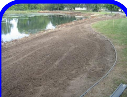
Seed bed preparation and installation of edging at project boundary
